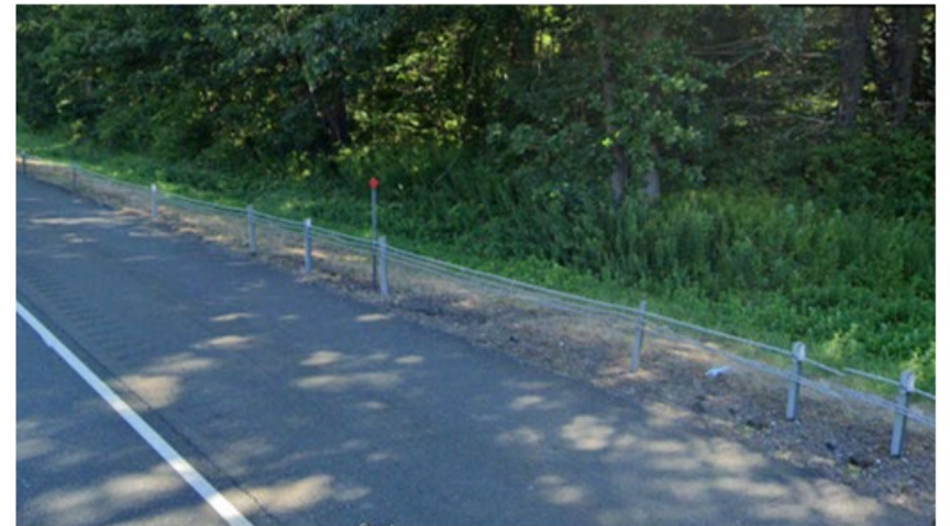
Example: Cable Guiderail with Steel Posts
